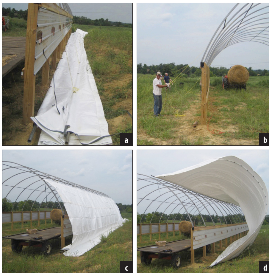
Figure 19. Setting up the nylon ropes to pull the tarp and pulling it into position.
