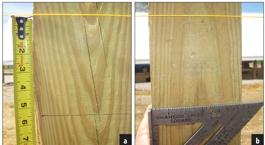
Figure 8. Measure down from the string line. Mark the bottom line using a speed square.
