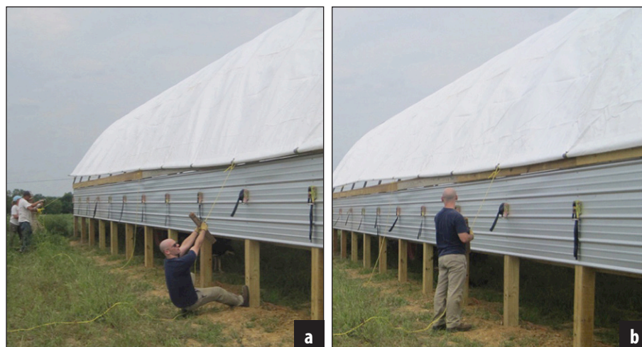
Figure 20. Leveling out the tarp along each sidewall to ensure ratchets will work.
