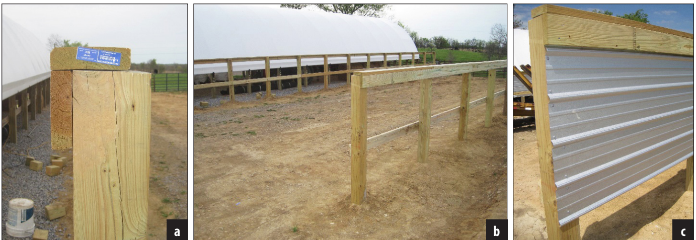
Figure 10. Treated 2 x 6 inch 12-foot-long fence boards are placed on the top of the knee wall and 36 inches up in the inside of the sidewall and screwed into each post. One run of metal siding was placed along each sidewall.
