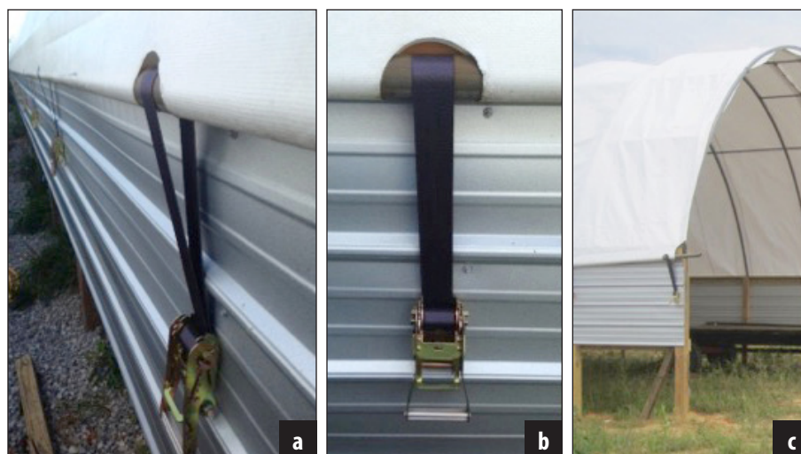
Figure 21. Ratchets to hold the tarp along the sidewall.
