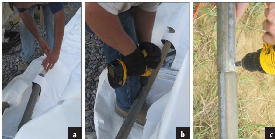
Figure 18. Feeding poles through the tarp along the sidewall and attaching pole pieces with self-taping screws.
