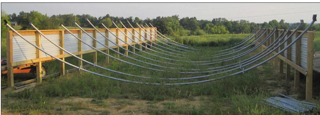
Figure 12. The ribs are set up in preparation for raising them above the knee wall.
