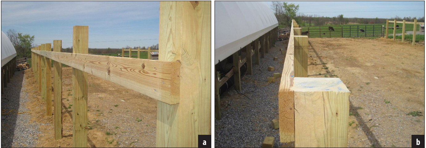
Figure 9. Treated 2 x 6 12-foot-long fence boards are placed above the marked line on the post and screwed into each post. The fence posts are cut off at the top of the 2 x 6.
