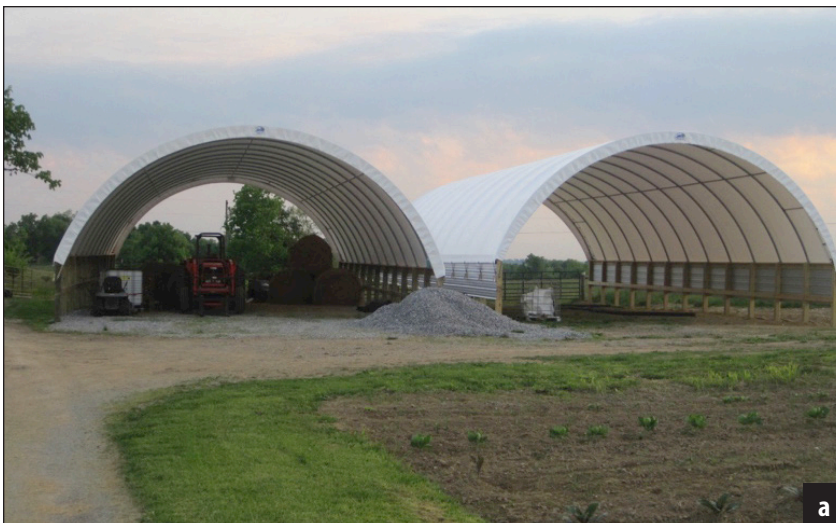
Figure 26. Preparing to spread gravel in the barn over filter fabric.
