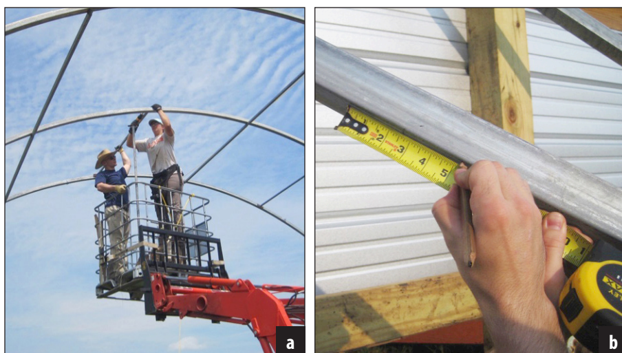
Figure 16. Adding additional cross bracing between the outside two ribs and marking these locations on the ribs.
