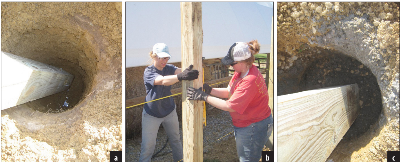
Figure 5. Anchor the posts with prepared concrete. Ensure that the posts are upright and properly spaced. Backfill the post hole with soil.
