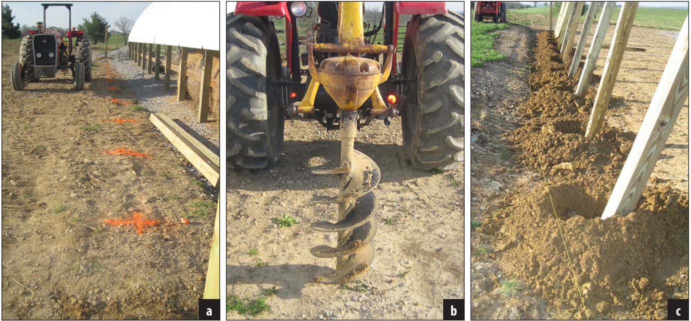
Figure 4. Mark locations for the posts along the sidewall. Dig the holes with an auger. Place the posts in the holes.
