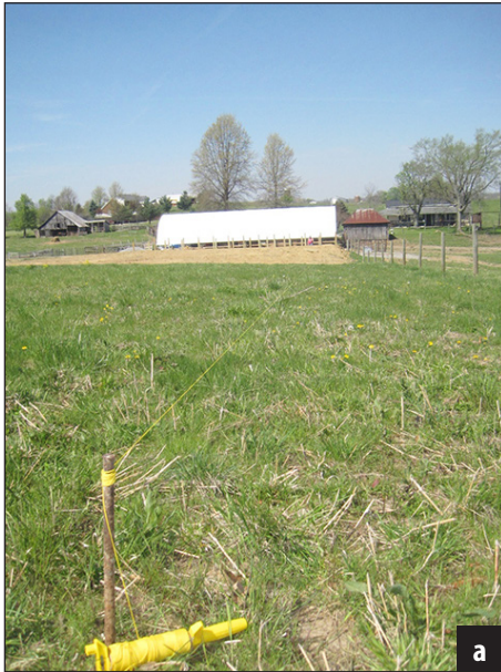
Figure 2. String lines for the hoop barn.
