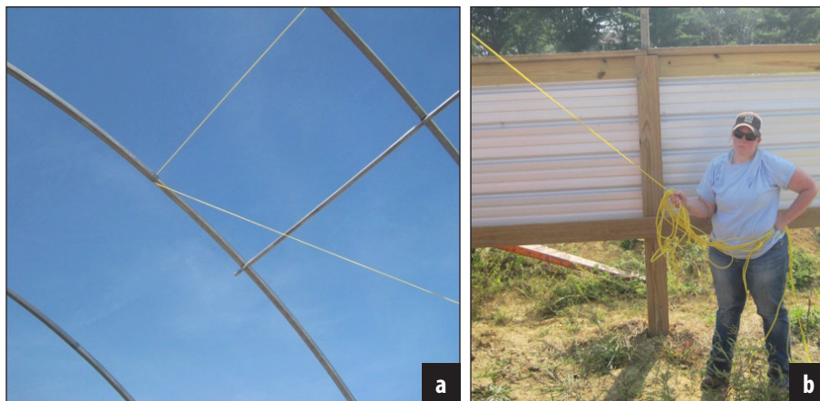
Figure 15. Using rope to stabilize ribs while the ribs are being mounted to the knee wall.
