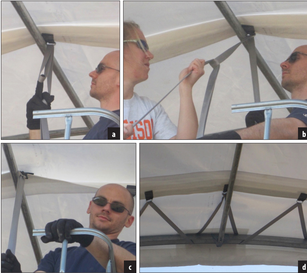
Figure 23. Beginning to lace the tarp along the end starting from the center at the top of the hoop.
