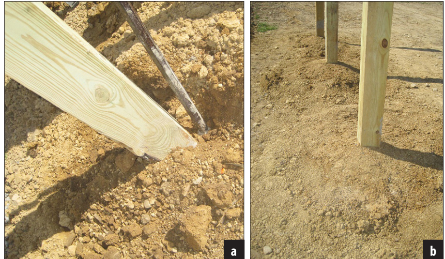
Figure 6. Tamp the soil down with a digging iron. Mound the dirt around the post for extra stability and to divert water away from the post.
