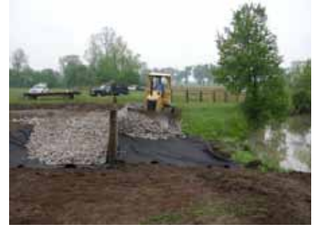
Figure 8. Rocks are pushed up on both sides of the posts to collect soil runoff and filter water before it reaches the stream. Rocks also give newly established vegetation something to cling to.
