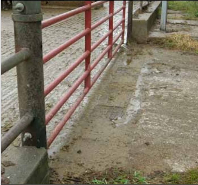
Figure 5. Clogged driveway grate that allows a discharge from the production area.
