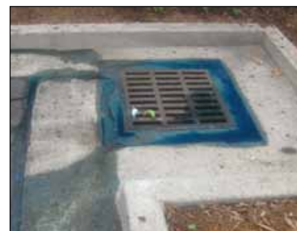
Figure 3. Unidentified blue substance flowing into storm drain located at the edge of a parking lot.
