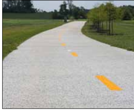
Figure 5. Permeable pavement, a good option for walking paths and trails, was used on part of the Legacy Trail in Lexington, Kentucky.
