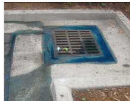
Figure 3. Unidentified blue substance flowing into storm drain located at the edge of a parking lot.
