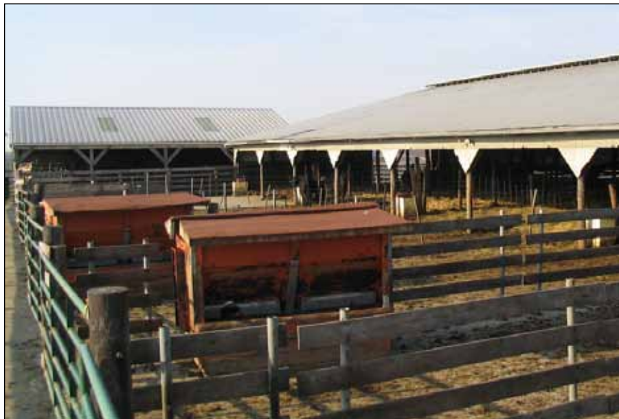
Figure 2. A typical paved feeding area with a guttered roof to redirect clean water away from the production area.
