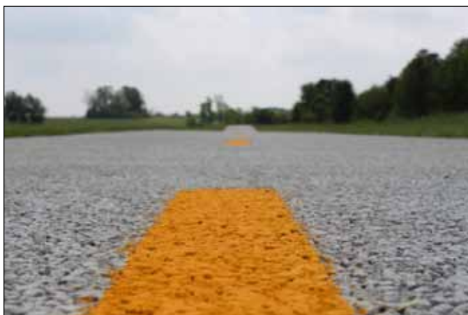
Figure 4. Pervious concrete was used to construct a portion of the Legacy Trail in Coldstream Park in Lexington, Ky.
