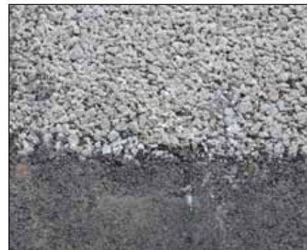
Figure 2. Permeable pavement (upper portion of figure) has large void spaces to allow water to infiltrate, unlike traditional asphalt (lower portion of figure).
