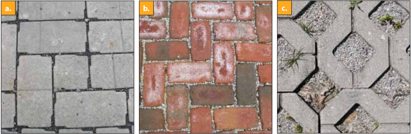
Figure 6. (a) Permeable interlocking concrete pavers (PICP), (b) permeable interlocking clay brick pavers (PICBP), and (c) concrete grid pavers (CGP).
