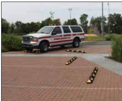
Figure 1. Used to construct the parking spaces (permeable pavers), sidewalks (pervious concrete), and roadways (porous asphalt) at the fire department in Georgetown, Ky., permeable pavement allows stormwater to infiltrate to the underlying soils.
