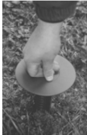
a. Installation of the Sentricon station.
