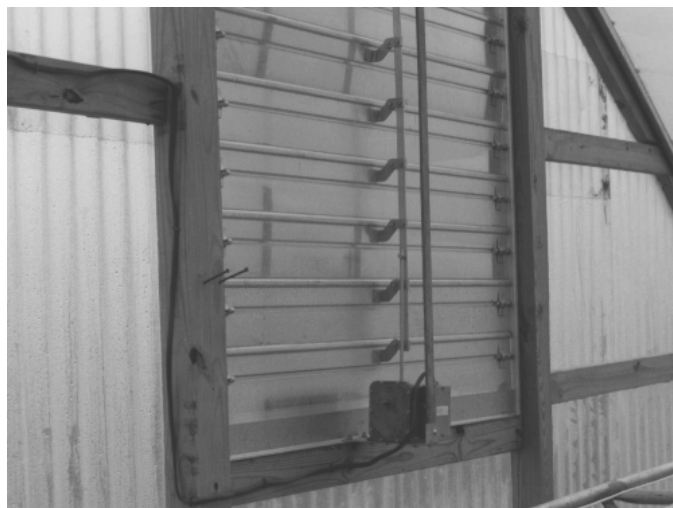
Figure 16. Motorized inlet shutter.
