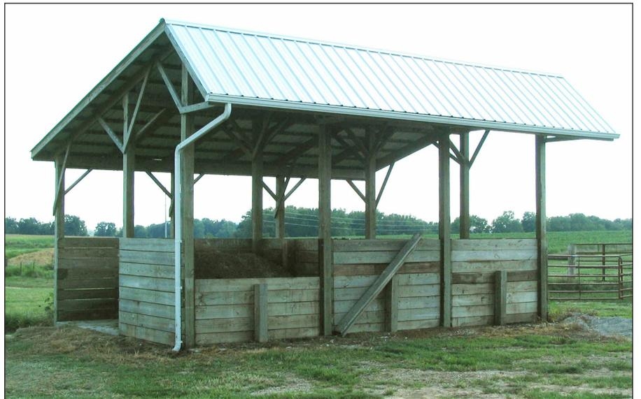
**Figure 5.** A three-bin shed with roof and doors.
