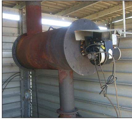
**Figure 2.** An afterburner used for a more efficient burn of exhaust gases.
