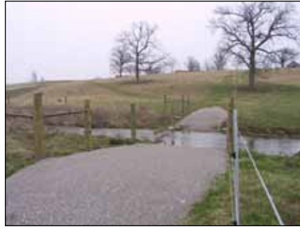
Photo 2. Stream crossings limiting livestock access to the stream. Courtesy of Carmen Agouridis and Jose Bicudo.
