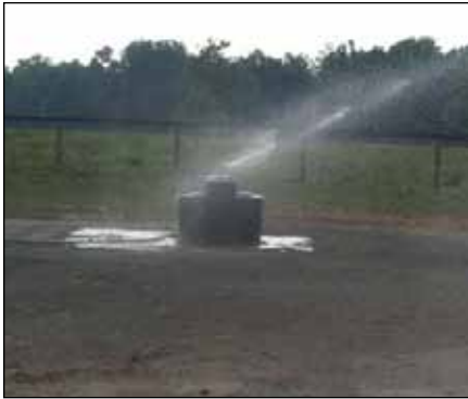
Figure 3. A 360-degree sprinkler is one way to keep the soil-cement wet.
