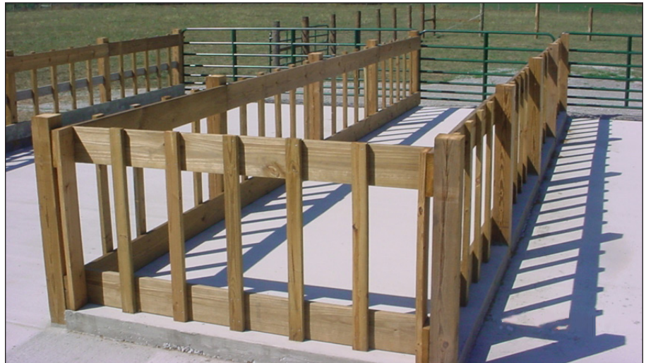
Figure 1. This winter feeding structure protects pastures, reduces labor, and decreases costs.
