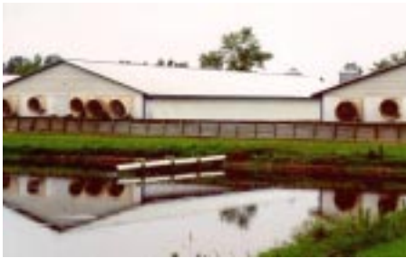
A lined earthen basin is an appropriate storage structure for liquid manure.
