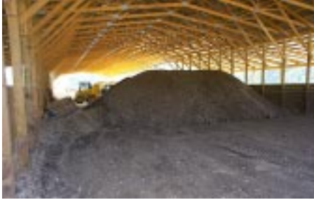
A covered structure provides manure storage until the appropriate application time.
