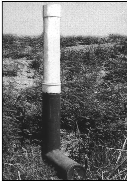
Figure 3. Outside drain fitted with a "T-stand pipe" and alfalfa valve.
