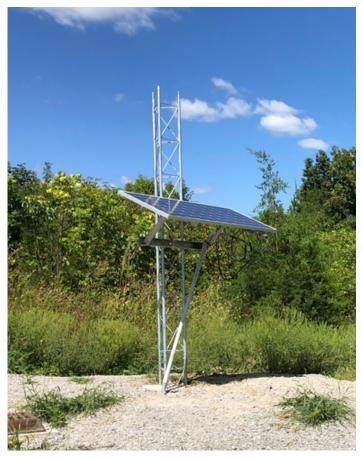
**Figure 7.** A solar-powered pumping system is a useful tool for remote locations. This one is used to pump collected water to a livestock waterer located 275 feet away and 40 feet higher in elevation. The iron grate in the foreground covers the catch basin.
