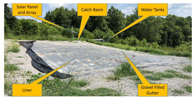
**Figure 5.** The rain trap area after construction, during which the brush and trees were removed and the land was graded to create the final surface for the trap. In the background is the solar panel and array used to power the water pump system. The top of the water tank, which stores a portion of the collected water, can barely be seen. A second water tank was added the following year.
