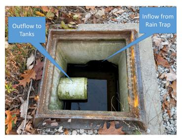
**Figure 6.** A catch basin collects the flow in one location, provides a chance for sedimentation to occur, and transfers the collected water to storage. The catch basin also includes a trash grate, which was removed for the photo.
