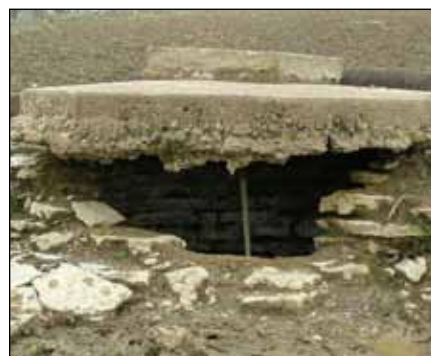
Figure 3. This abandoned well is located in an agricultural area that is void of vegetation that could filter pollutants from stormwater runoff and reduce the amount of pollution entering groundwater resources.
